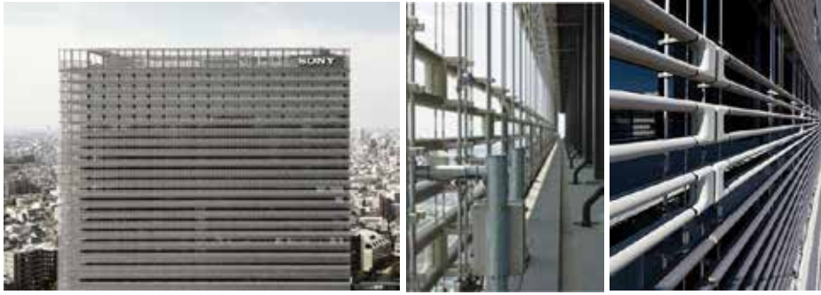
Figure 13 South elevation detail of Sony City Osaka
