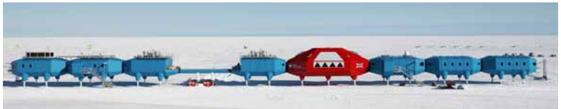
Görsel 12: Halley VI British Antarctic Research Station - Kaynak: https://bbarchitects.co.uk/halley-vi-british-antarctic-research-station/
